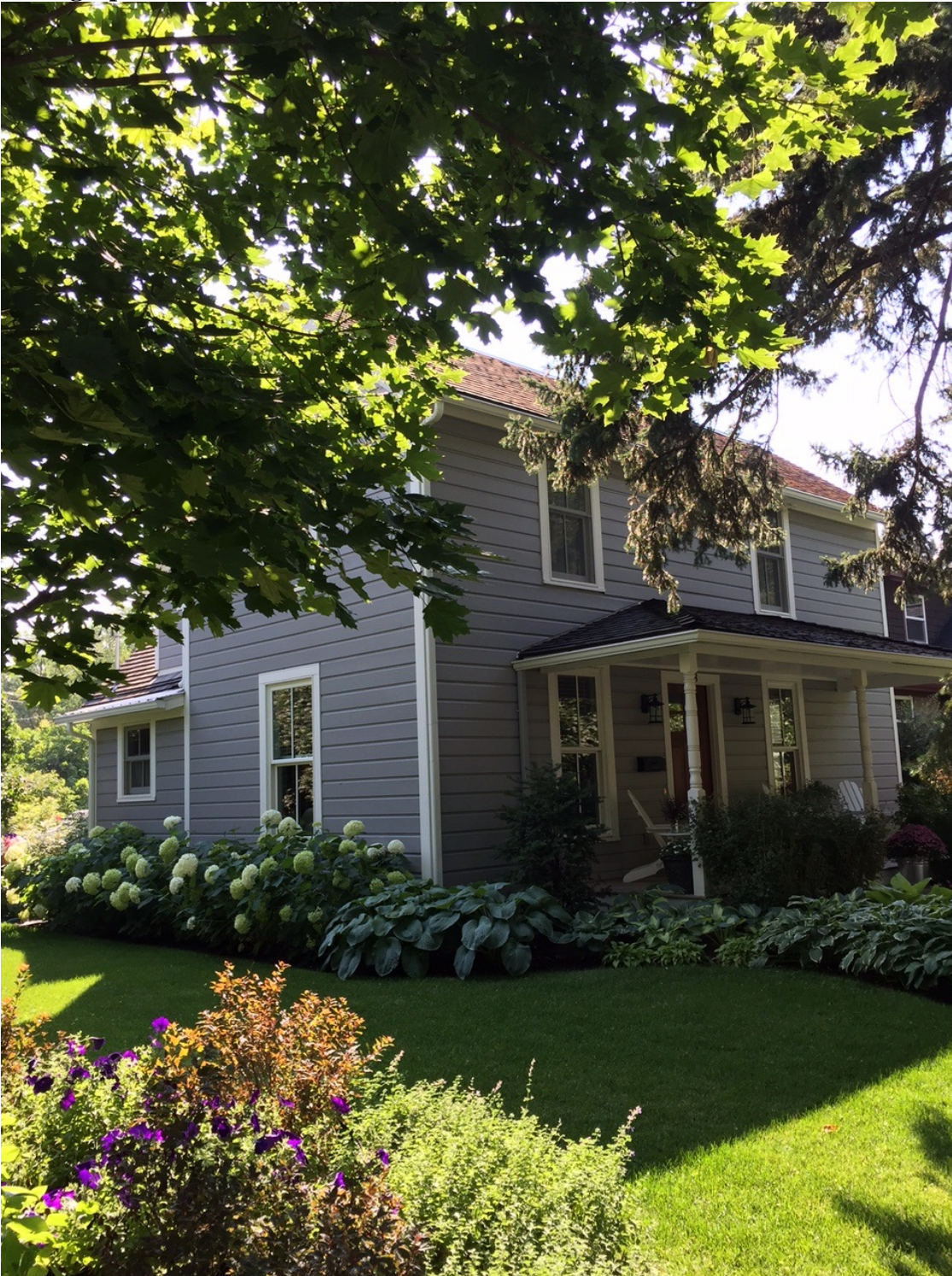
McDonald House View of West Façade and partial north elevation, facing southeast Photo taken 8/30/15, by Crystal Alegria
