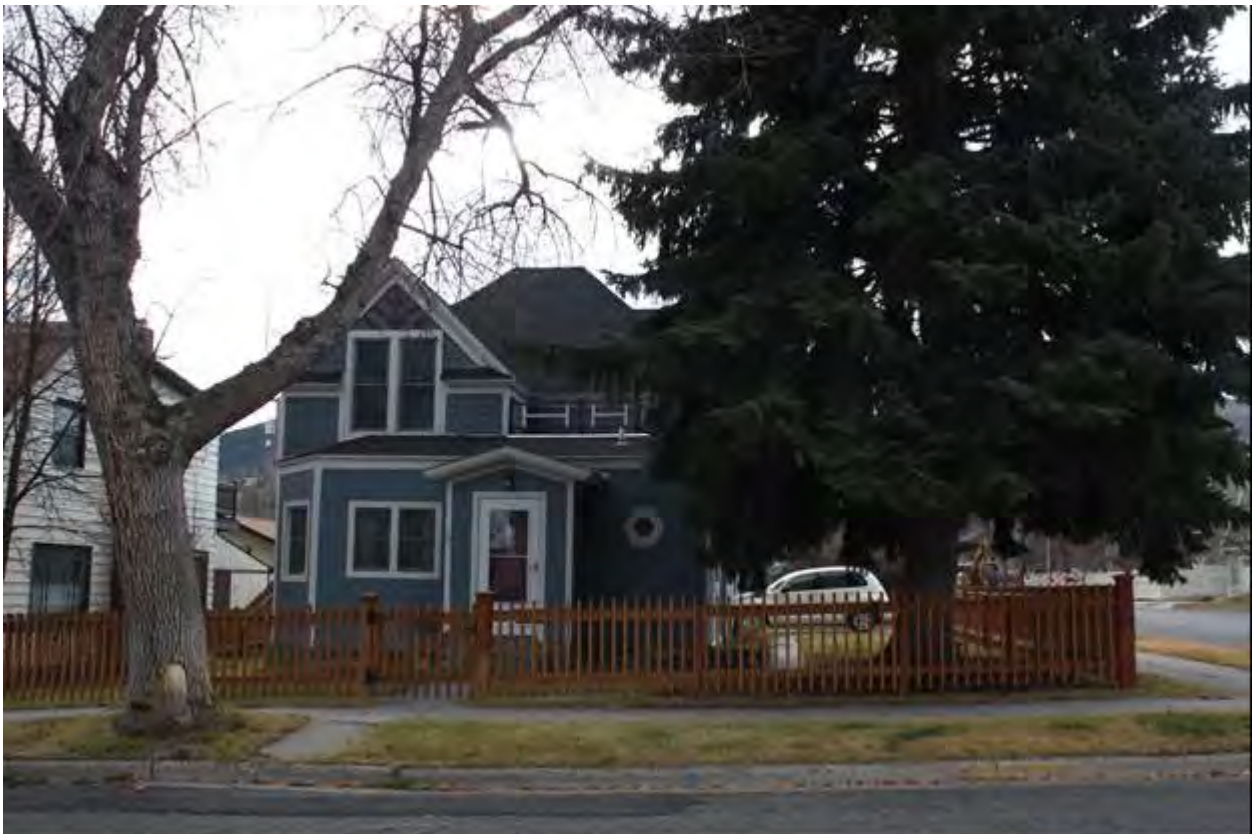
MT_LewisAndClarkCounty_Crump-HowardHouse_0001, Main House, overview, view to S.
