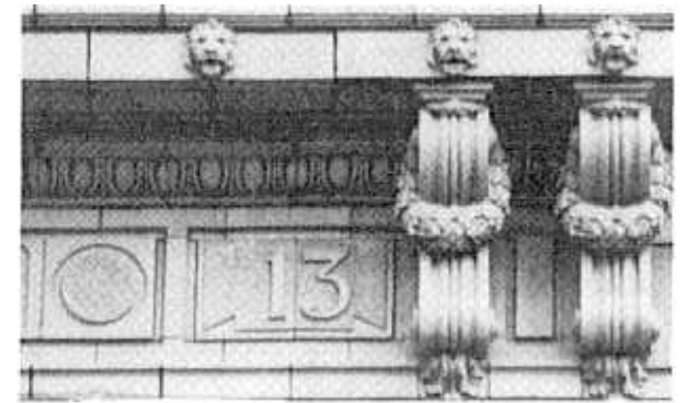
9. The narrow three story richly decorated facade of the Warr Lane Building makes elaborate use of terra cotta and the polychrome brick. Note the central cartouche "skylined" on the entablature capping the building, and the eight antefixa (lion's heads) just below. Built in 1913, the building was designed in the Beaux Arts style by the local office of architects Link & Haire.
