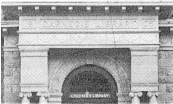
The Carnegie Library was designed and built by T.J. Tubb, an early contractor. Built in the Roman Revival style popularized by Thomas Jefferson, it features many of the design idioms of that style, namely the raised platform, the four columned portico with pediment enclosing an arch or lunette.
