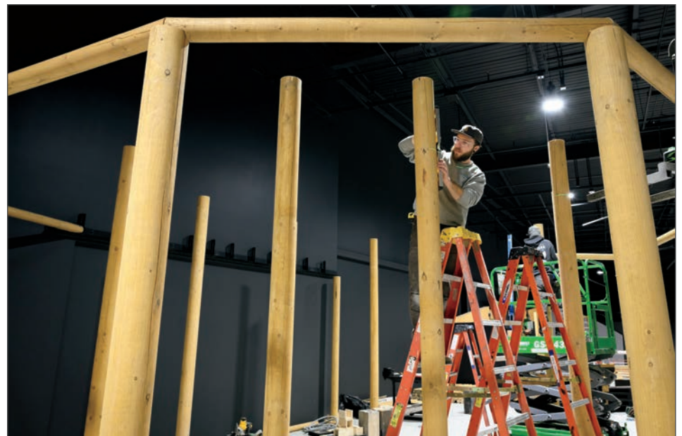
A Cinnabar crew member levels the poles that form an arbor in the Sovereign Nations zone of the Montana Homeland Gallery.
