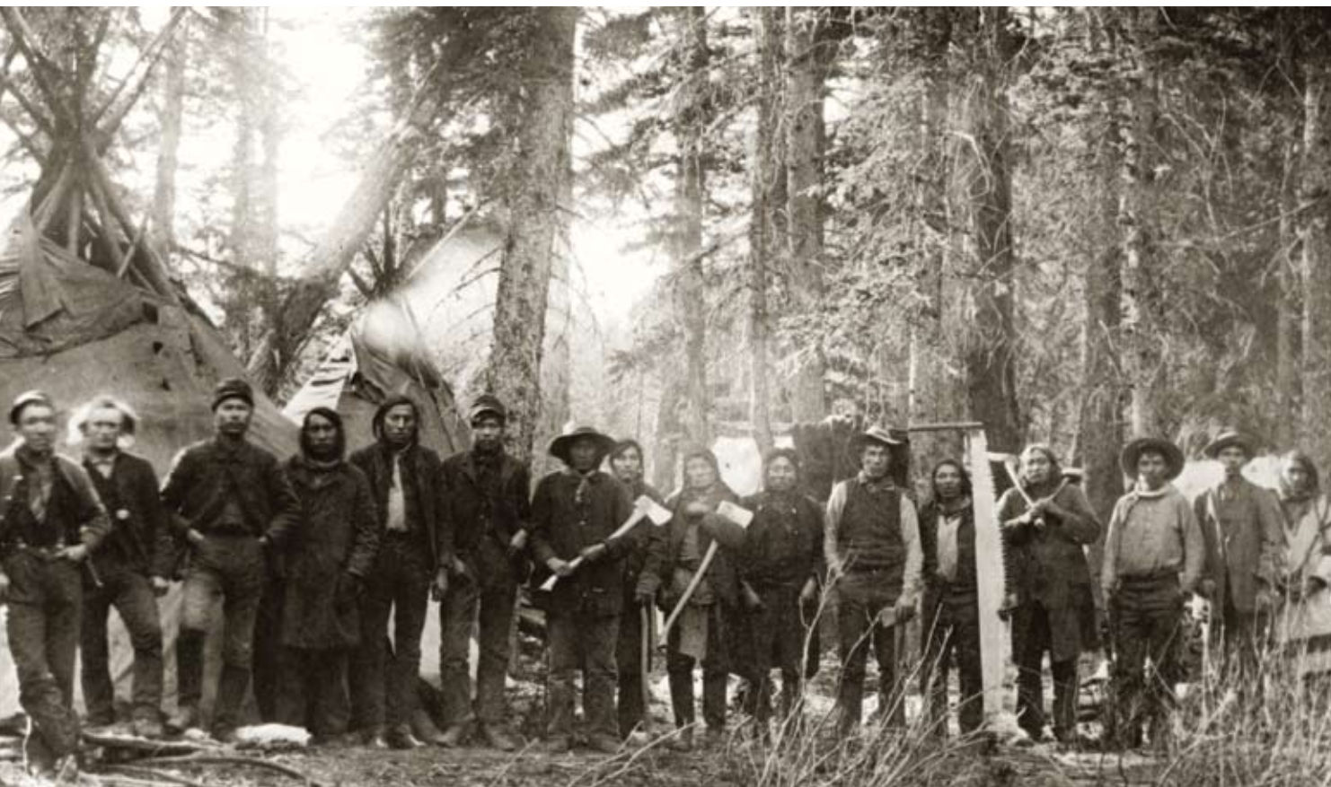
FIGURE 18.10: Indian Civilian Conservation Corps crews, like this Blackfeet logging and forestry crew, provided needed jobs on the reservation.
