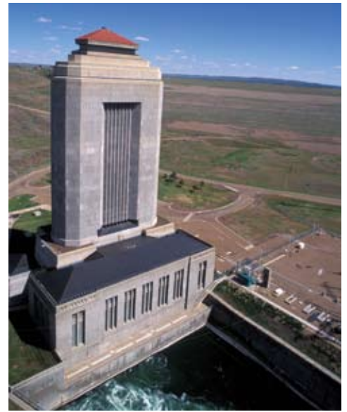
FIGURE 18.11: The Fort Peck Dam was an immense example of American muscle and engineering know-how. It immediately became a symbol of America’s recovery from the Great Depression.
