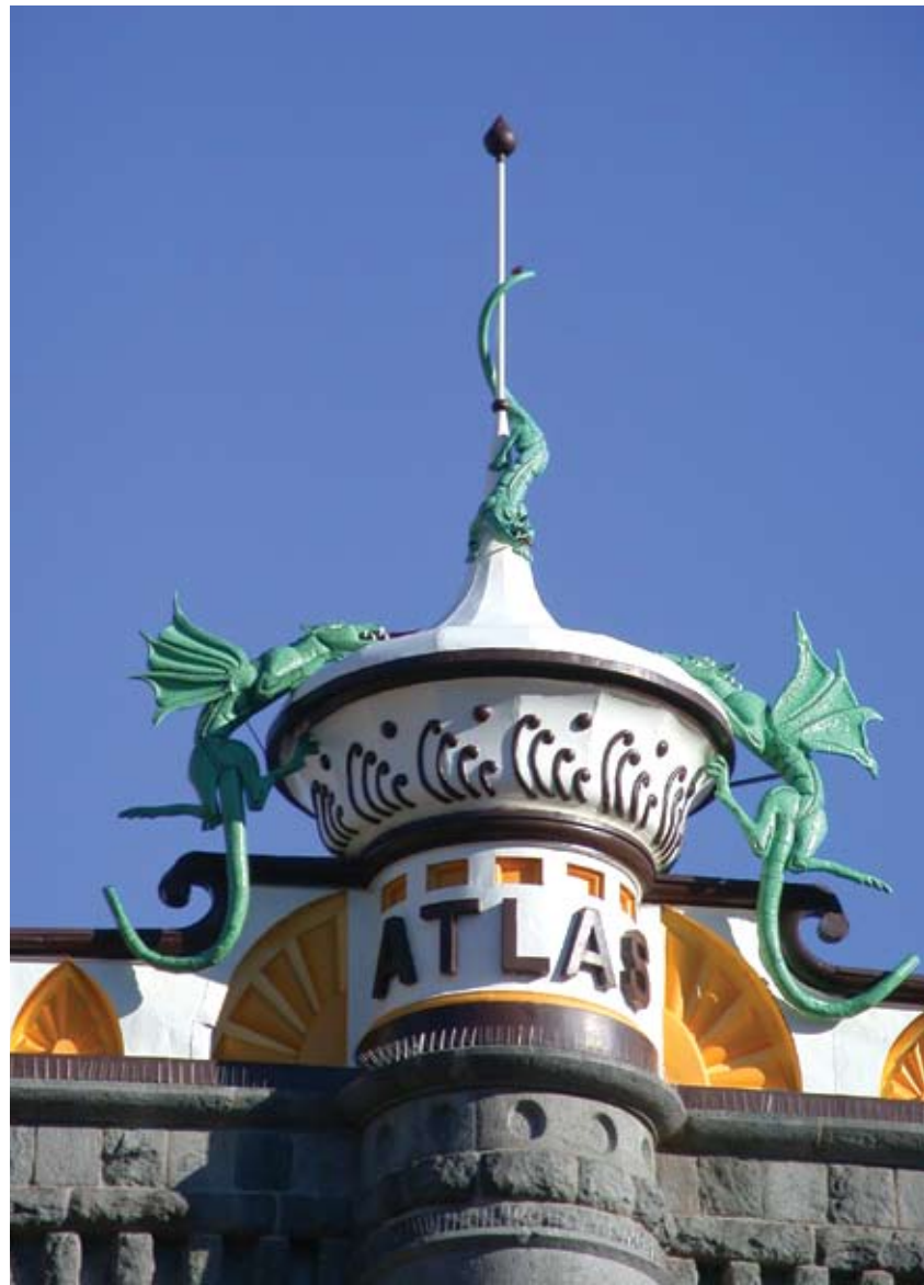
FIGURE 14.13: To learn more about your town, look up. Architectural details around doorways and windows and at the top of buildings tell you something about the craftsmen in your community. When people were proud of their buildings, they added special touches to make them look more interesting or impressive.
