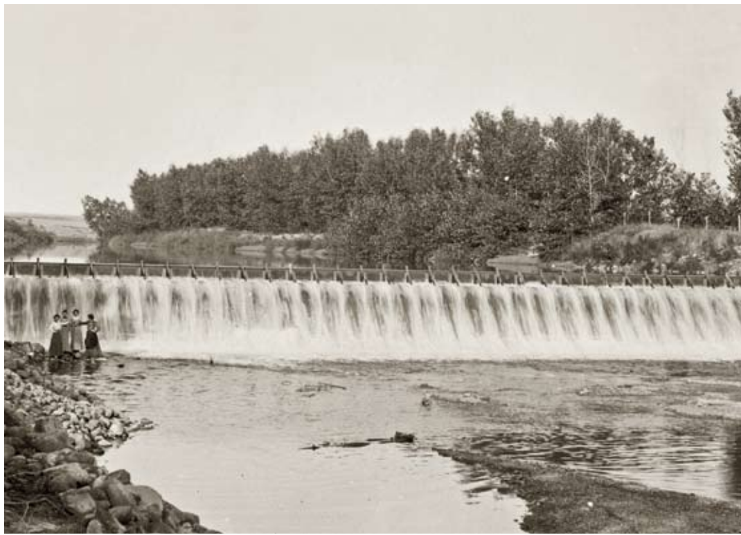
FIGURE 11.12: The Fort Belknap tribes built this dam across the Milk River to supply water to reservation farmlands. But upriver settlers took so much water that there was not enough left for the reservation. Ultimately, the U.S. Supreme Court upheld the tribes' water rights.
