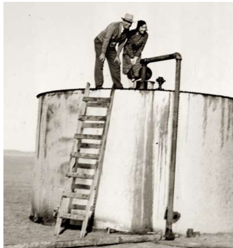
FIGURE 11.15: Oil discoveries in northern Montana made companies very interested in drilling for oil on Blackfeet land. These two people are watching the tank fill up with the first commercial production of oil from an oil lease site on the Blackfeet Reservation.
