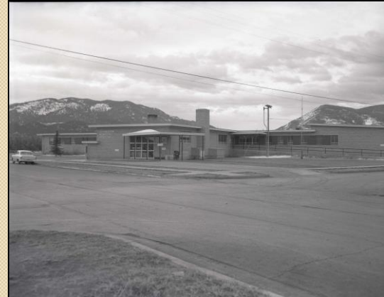
LIVINGSTON MEMORIAL HOSPITAL, PARK COUNTY, LIVINGSTON
