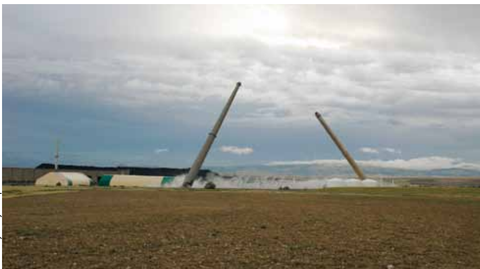
The Asarco smelter stacks in East Helena crashing down into history.
