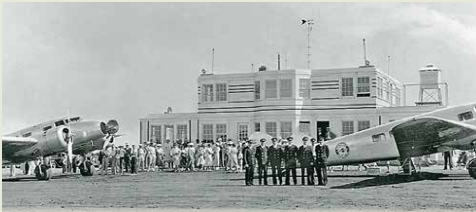
“New Hangar at Billings Airport,” 1937, MHS PAC 2006.5-7
