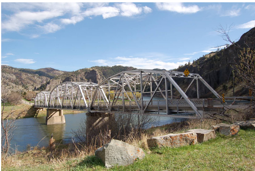
Hardy Bridge, Cascade County
