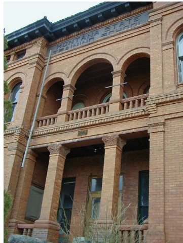
Historic Montana School for the Deaf and Dumb Administration Building, Boulder
