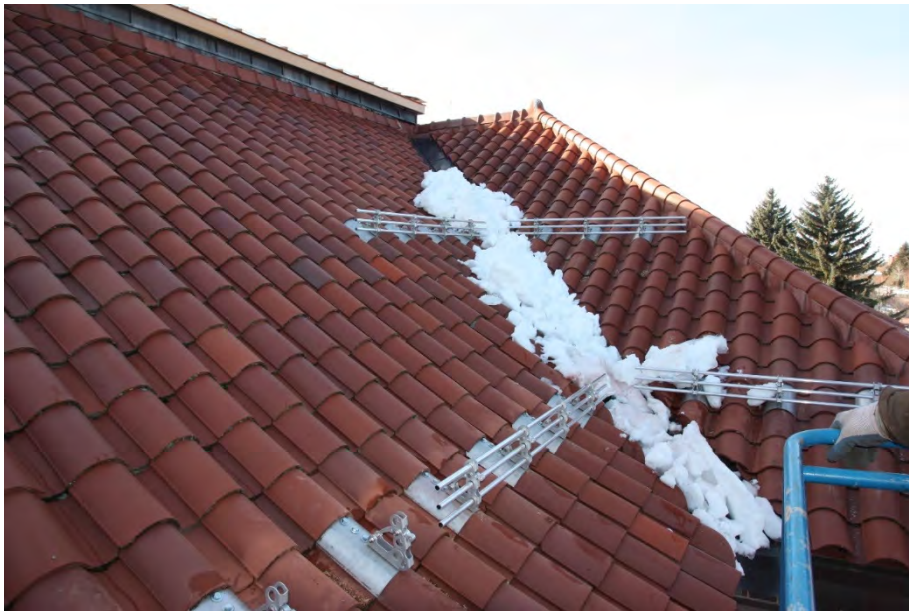
Figure 11: MSU-Bozeman, Roberts Hall during installation of snow guards. November 21, 2017.
