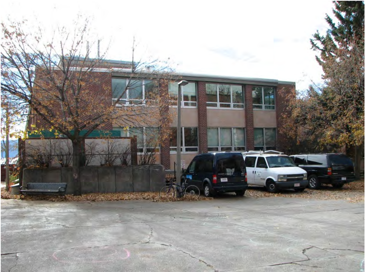
A.J.M. Johnson Hall North Elevation, Facing: S Montana State University Jessie Nunn, November 3, 2012
