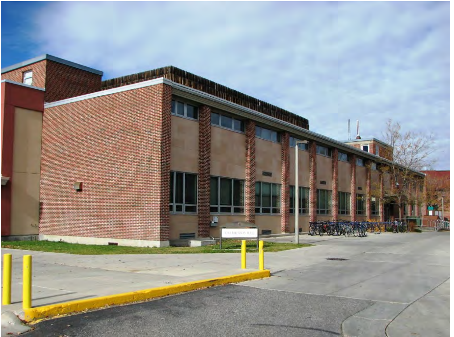
A.J.M. Johnson Hall East Elevation, Facing: NW Montana State University Jessie Nunn, November 3, 2012
