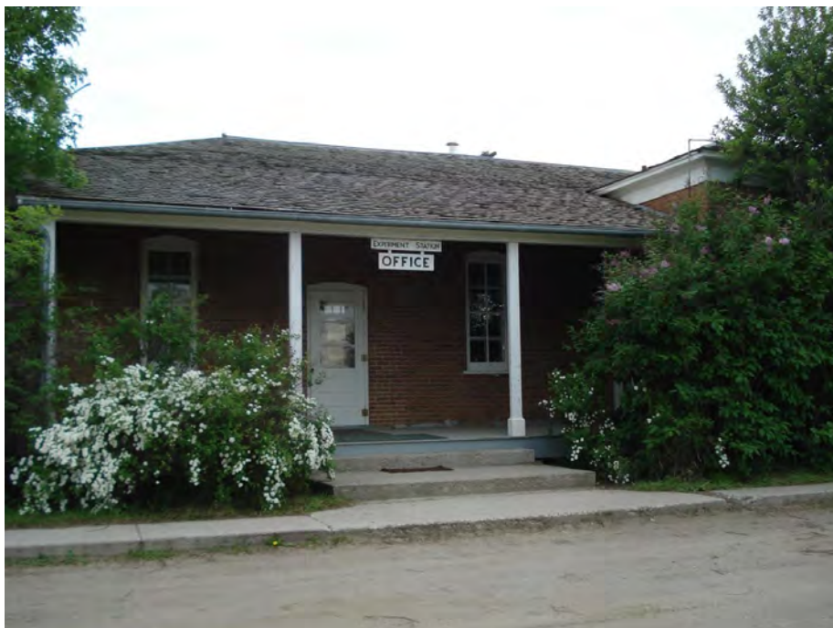
Figure 19: Fort Assiniboine, Post Library (c.1889), previously used for offices by NARC. The building is now vacant.
