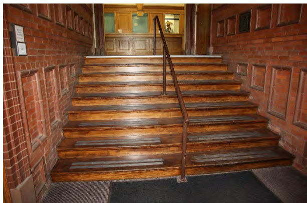
Figure 14: MSU-Bozeman, Montana Hall, interior north stair. May 12, 2017.
