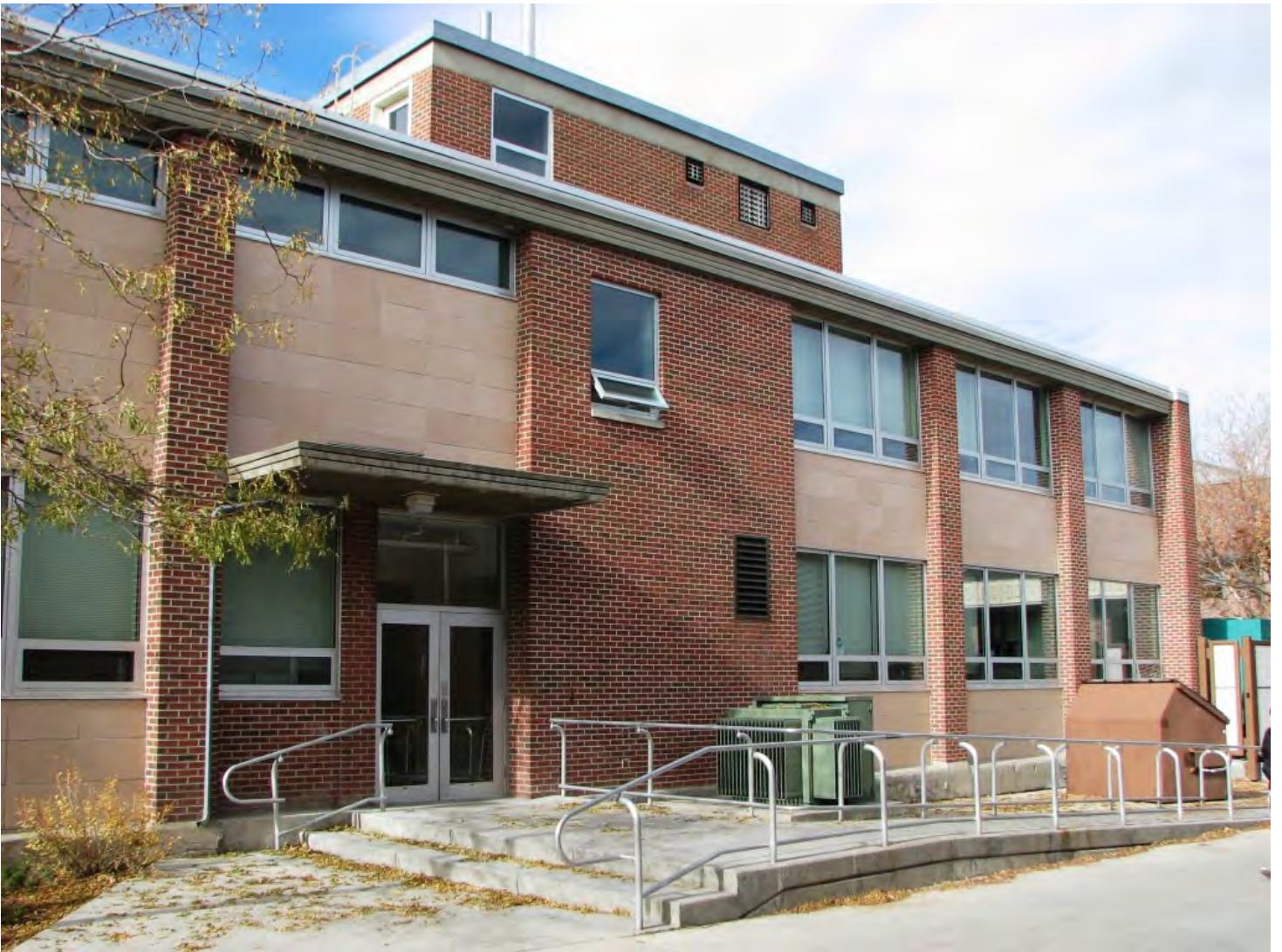
A.J.M. Johnson Hall East Entrance, East Elevation, Facing: NW Montana State University Jessie Nunn, November 3, 2012
