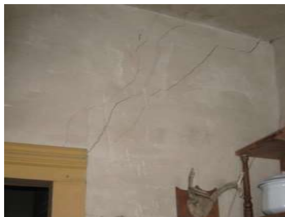
Cracked plaster
