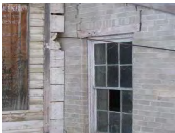
Cracking brick
