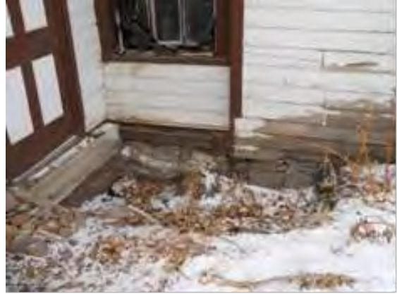
Failed foundation
