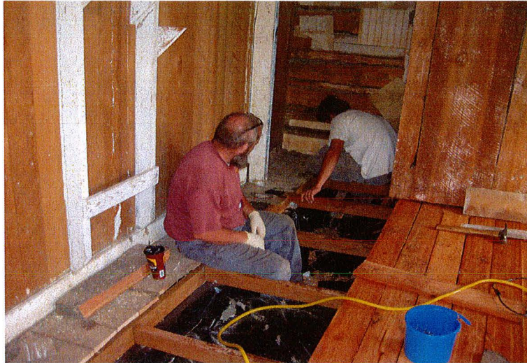
Figure 4. Replacing flooring at the Parsonage, Bannack State Park/NHL.
