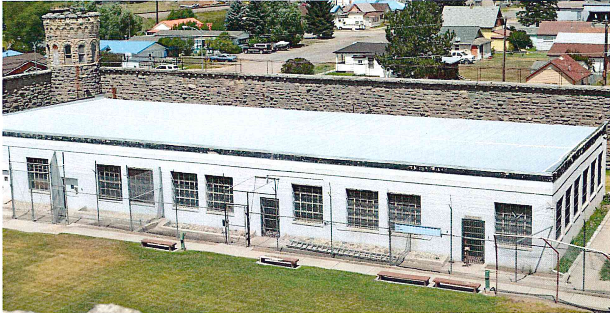
Administration Building – Old Roof
