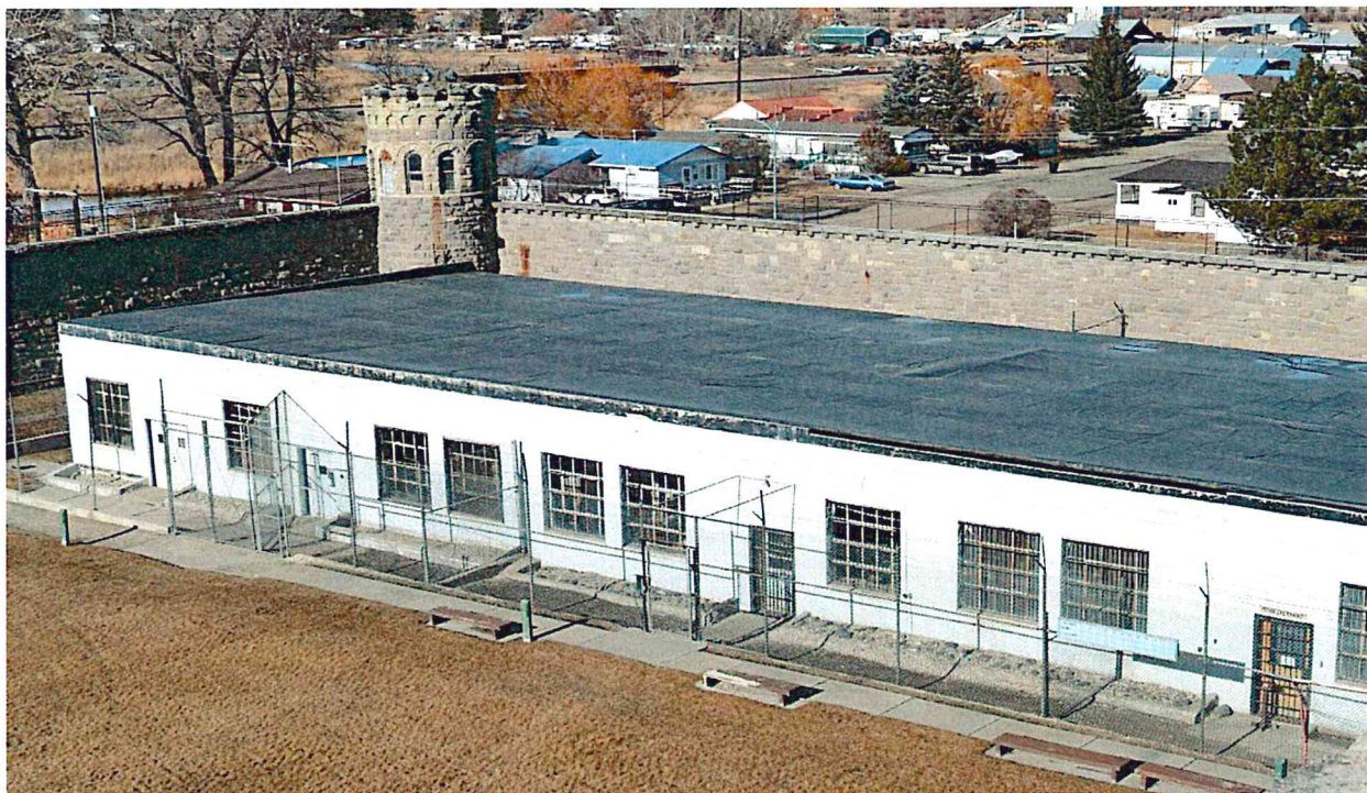
Administration Building – New Roof 2019
