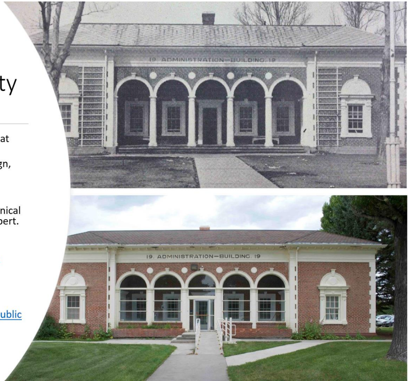
Warm Springs Administration Building
